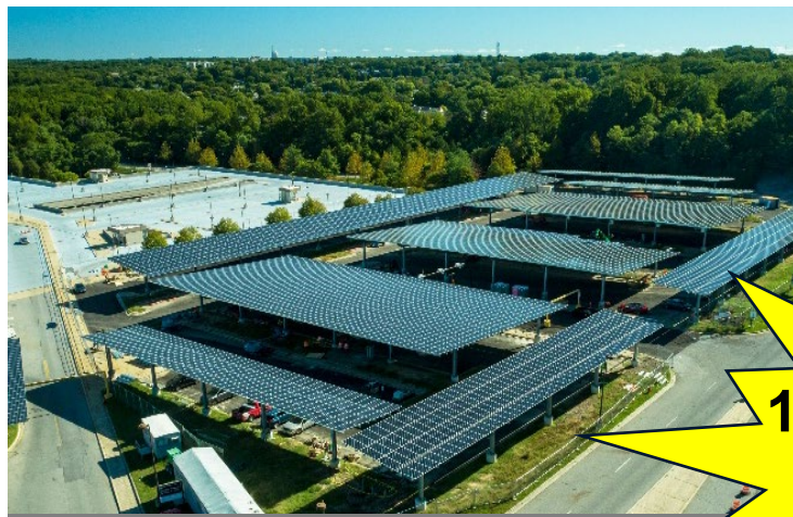
Southern Avenue Station
