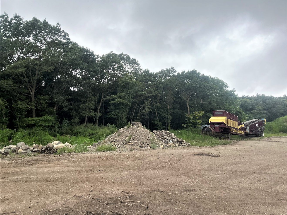
Photograph No. 1: Exterior view of Sample Plot SP-3 edge habitat and site operations, facing northwest (July 14, 2023).
