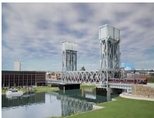
9 WALK Bridge Replacement
