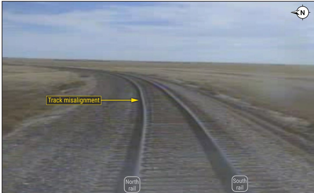
Figure 4. Still frame from Amtrak Train 8 that shows the misaligned BNSF track.
