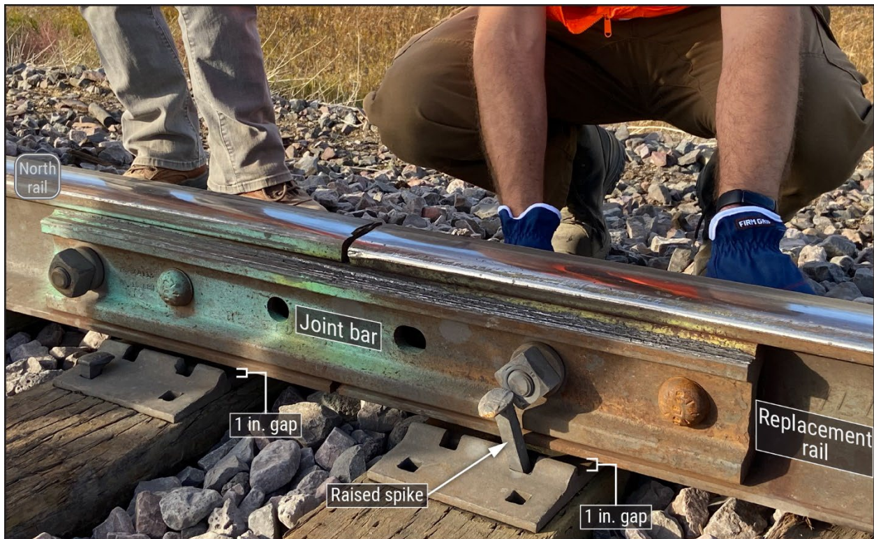
Figure 14. Photograph of a bolted replacement rail.
