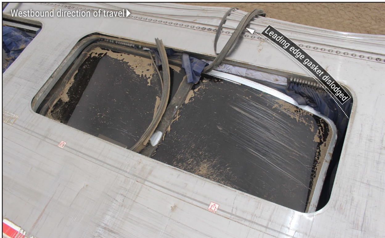
Figure 11. Exterior photograph of a window from Railcar 9.
