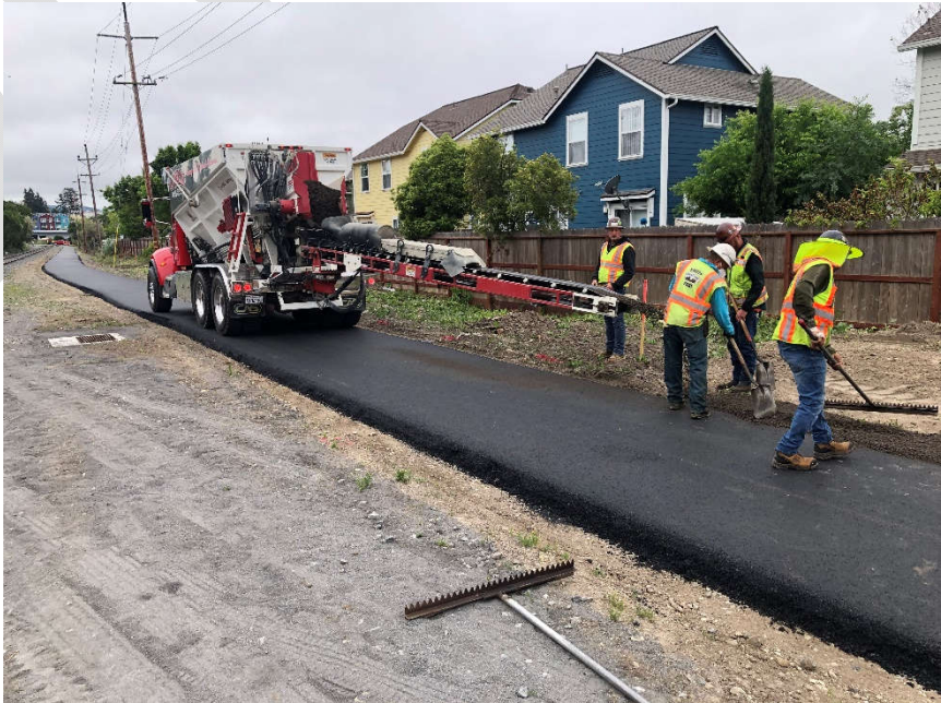
Payran to Lakeville Pathway Project
