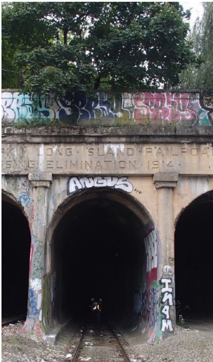
The East New York Tunnel, constructed over 100 years ago, would be rehabilitated for IBX service.
