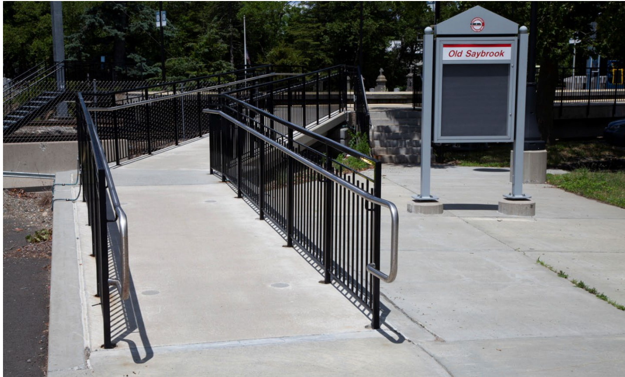
Figure 5-5. Accessible Pedestrian Ramp in Old Saybrook
