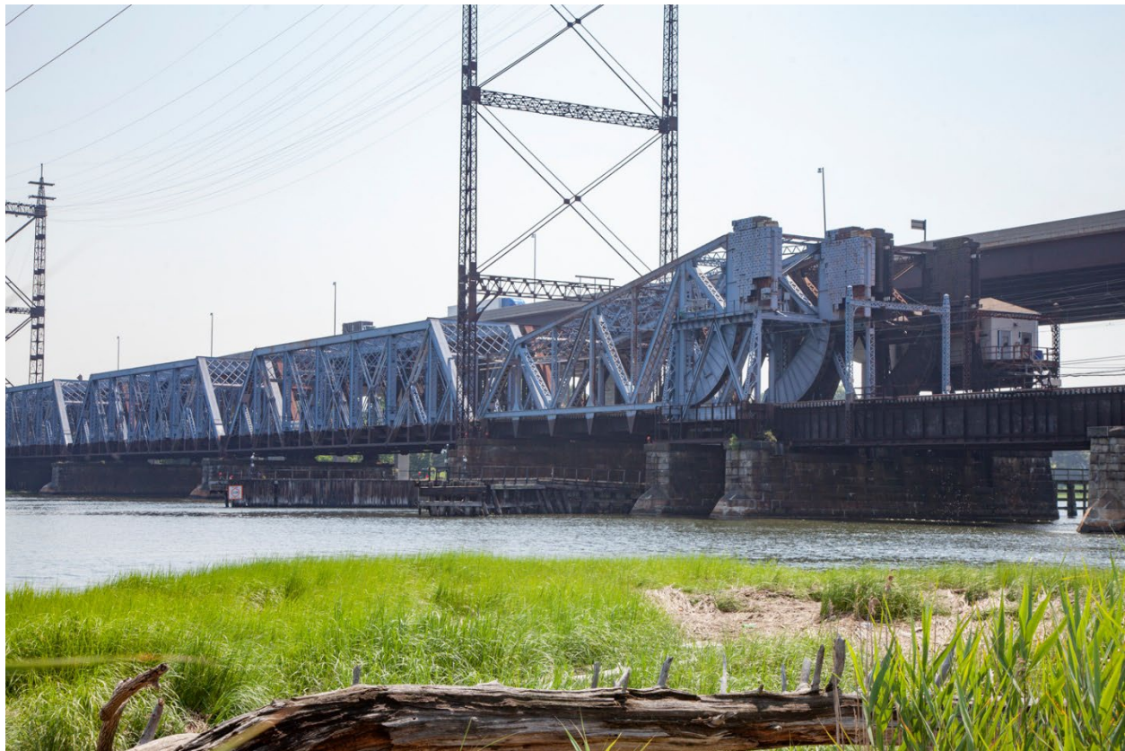
Figure 3-9. Existing Devon Bridge
