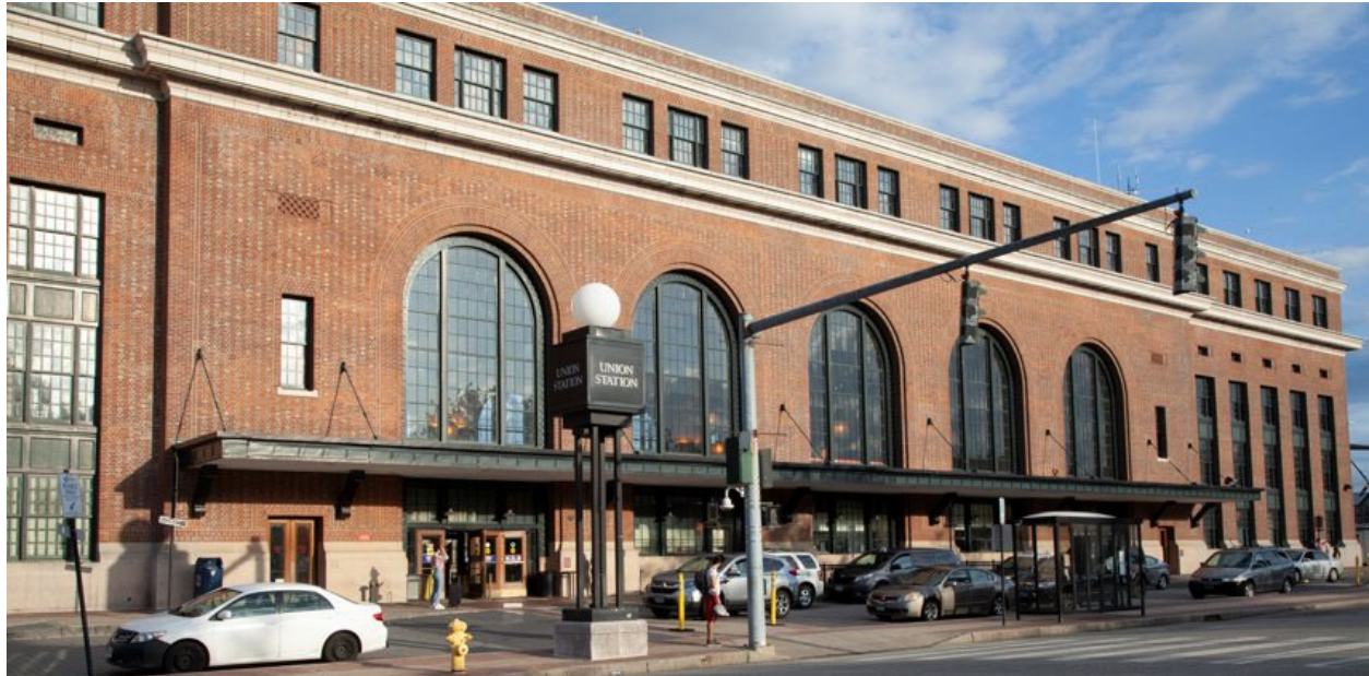
Figure 2-14. New Haven Union Station
