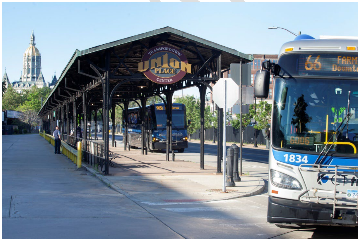
Figure 2-17. Hartford Union Station Transportation Center
