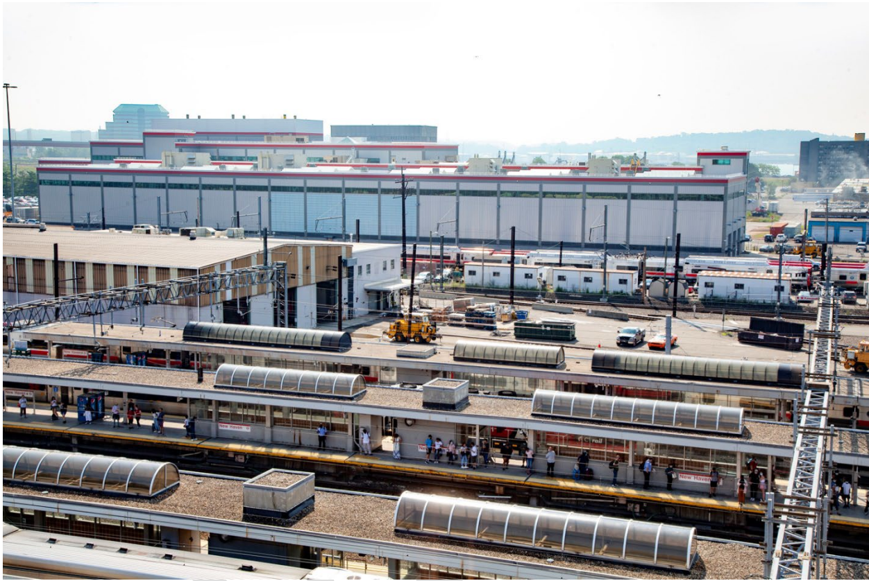
Figure 3-5. New Haven Yard Facilities
