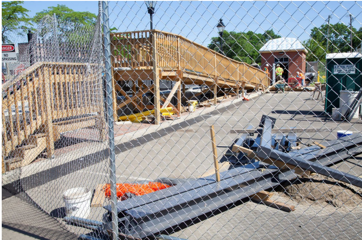
Figure 5-2. Temporary ADA Ramp Construction at Windsor Station (Construction Complete in July 2022)
