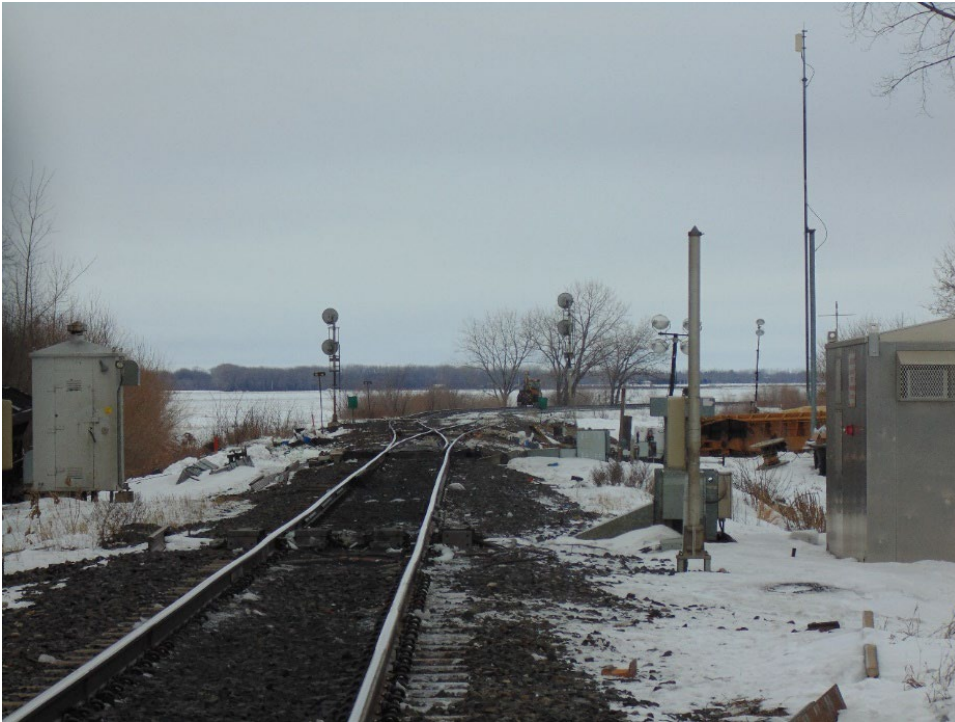
Figure 8. View looking westward of signals 504S and 504N at Nattress showing the transition from double to single main track (Source: TSB)
