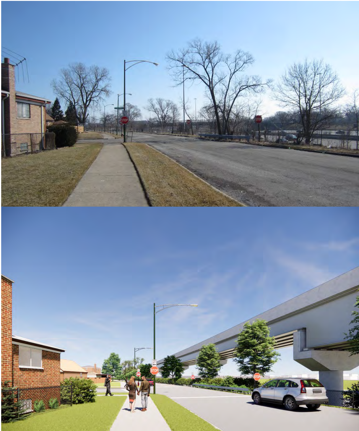
Figure 4-8: Existing Conditions and Photo Simulation of the Elevated Structure North of I-57 (Looking East from 98th Place and Princeton Avenue)
