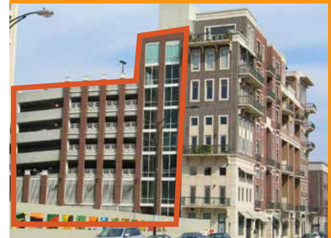
Top to bottom / 1 Raised stoop entries for housing at Glenwood Park, Atlanta, GA / 2 'Bookend' apartment concealing parking deck beyond, Greenville, SC
