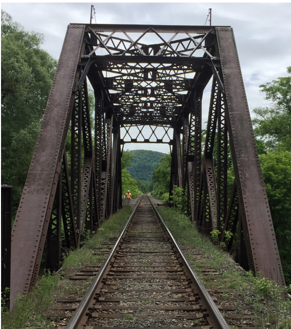
Hoosick River Truss in Pownal, New York.
