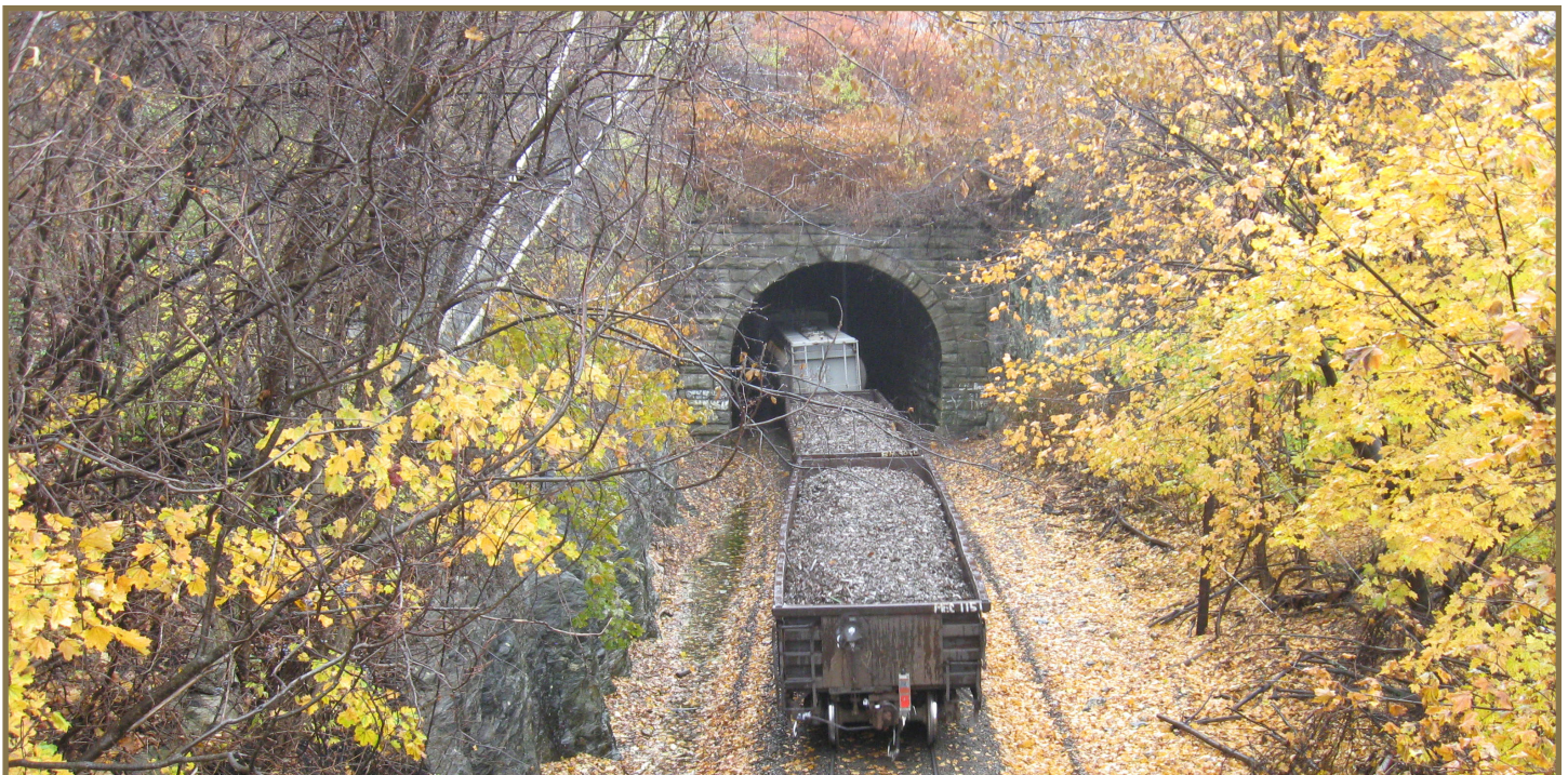
Little Tunnel in North Adams, MA.
