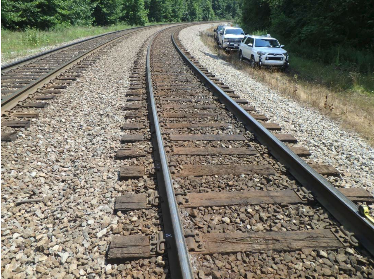
Figure 7. Accident curve facing east toward direction of accident train travel.
