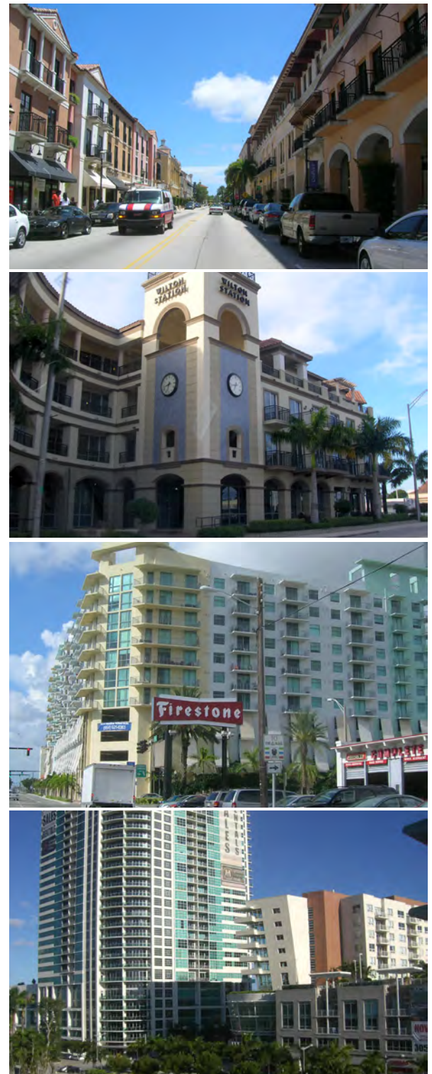
New mixed-use developments along the FEC corridor are of a higher density than surroundings and often take cues from the rail line. Top to Bottom: “City Place” in West Palm Beach, “Wilton Station” in Wilton Manors, “Hollywood Station” in Hollywood, and “Midtown Miami.”
