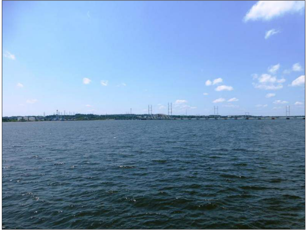
The Raritan River Drawbridge, as seen from the Sadowski Parkway Waterfront Park, looking west. Industrial sites are visible to the southeast but beyond the bridge to the southwest, only trees are visible 1
