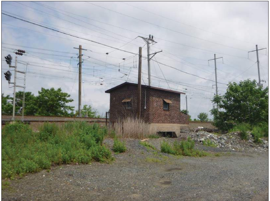
Electric Substation, a contributing resource to the New York and Long Branch Railroad Historic District (Map ID 3.1)
