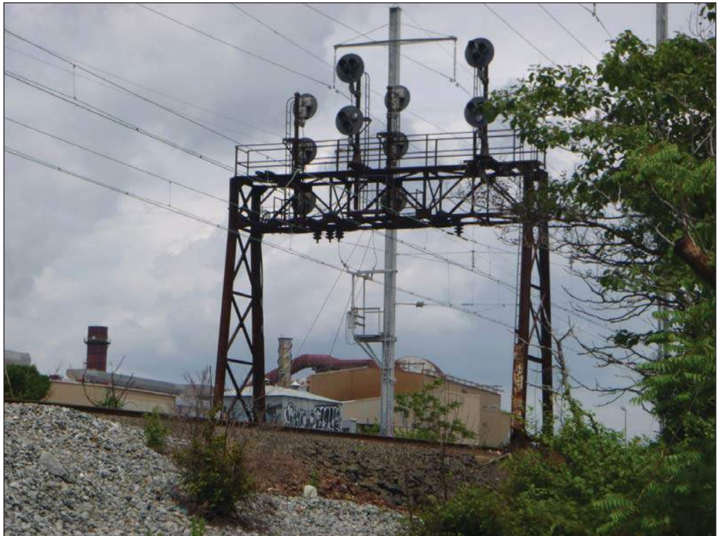
Railroad Signal Bridge, a contributing resource to the Perth Amboy and Elizabethport Branch of the Central Railroad of new Jersey (Map ID 4.1)
